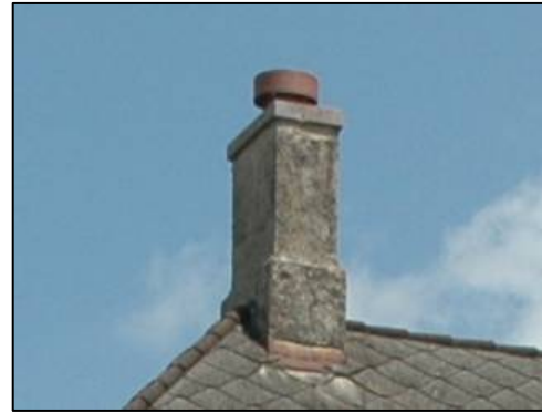
The coping and metal flue are character-defining features of this chimney.
