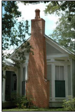
Note the tapered form of this brick chimney, along with the terracotta hood.
