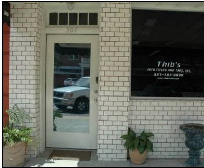
The character of an exterior wall is defined by its texture, color, and pattern. Note the use of glazed brick.
