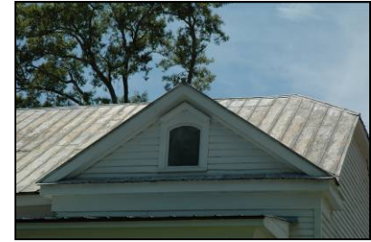
Note the standing-seam metal roof and the proportions of the primary roof and the gable end roof heights.
