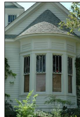
The geometric grid of muntins in this building's double-hung windows is a character-defining feature.
