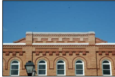
On this Romanesque Revival building, the parapet and cornice, with projecting brickwork, are important character-defining features.
