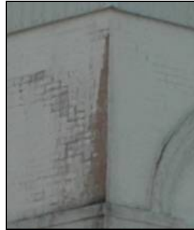
Note harder brick on the front façade and softer, secondary brick on the side façade or party wall, which requires gentle treatment if exposed.
