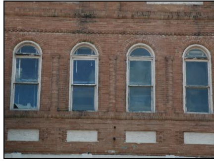
The projecting elements and treatment of the brick are character-defining features of the wall of this building.
