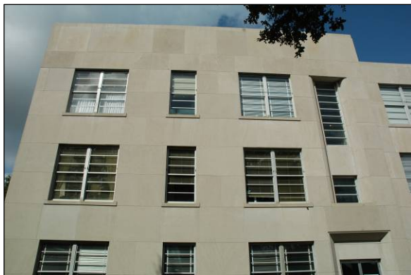
On a tall building, windows often compose the bulk of the main façade. These operable metal awning windows complement the verticality of the building.
