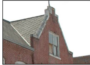
The brick parapet, stone coping, and diamond-shaped shingles, are all character-defining features of this Colonial Revival Style roof.
