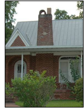
Note how this chimney projects beyond the exterior façade – the depth of the chimney is a character-defining feature that should be maintained.
